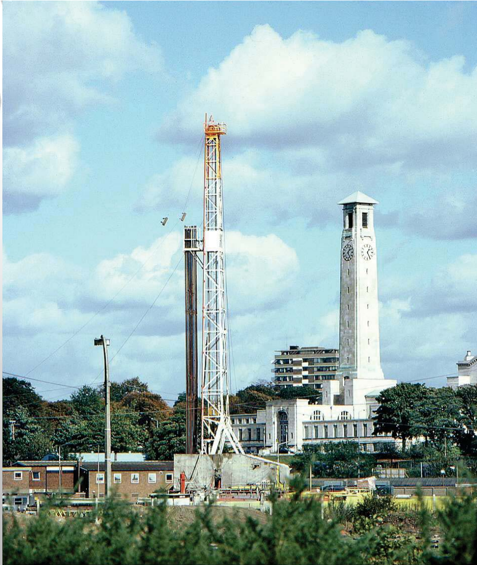
Southampton No.1 Geothermal Borehole in 1981. The target formation, the Sherwood Sandstone (Triassic) was encountered at 1729m., higher than expected. Thus, unfortunately, water at boiling point was not found. However, hot, concentrated brine at about 76 degrees C. has proved useful as a supplementary geothermal energy source. Ian West & Tonya West (c) 2008.
